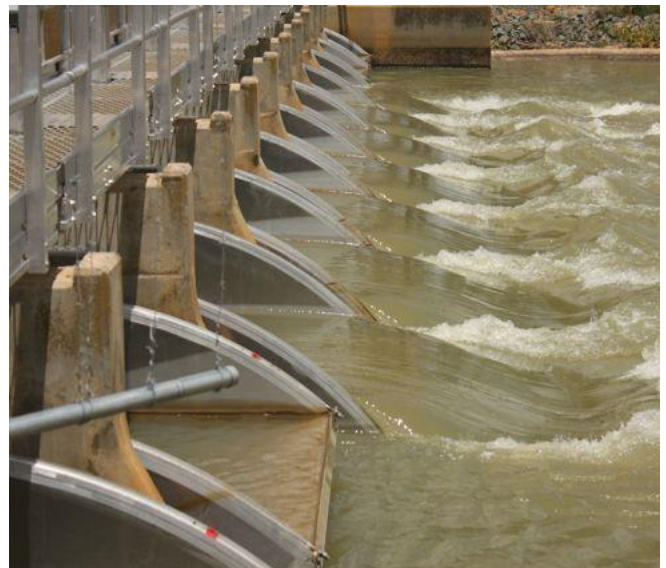
Figure 1 Water passing through flume gates along a channel.
